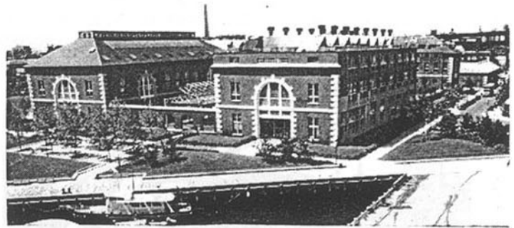
Fig. 2 Constitution Quarters (sub-buildings A & C)
