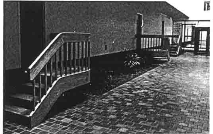
Fig. 15 Constitution Quarters Mall. Photo of ground-floor apartment entrance stairs and planter pits.
