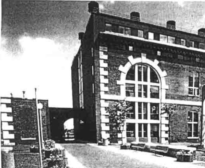
Fig. 13 Building 42C showing modifications to building, fragments of earlier structures, and easement.
